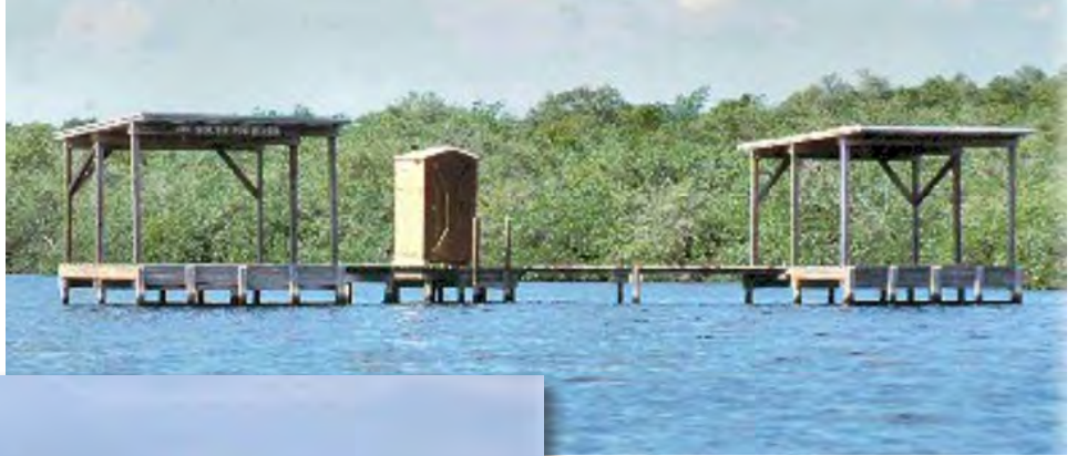
Docks with a shallow sloped roof supported by vertical posts with no wall structure. Source: Seaside Water Trail Camping Platform Feasibility.
