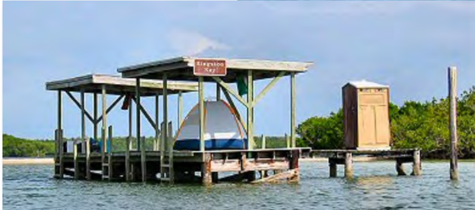
Docks with a shallow sloped roof supported by vertical posts with no wall structure. Source: Seaside Water Trail Camping Platform Feasibility.
