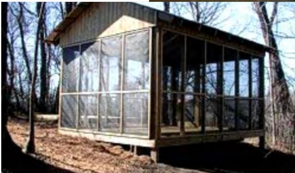
Example of Land Camping Structure. Source: Seaside Water Trail Camping Platform Feasibility.
