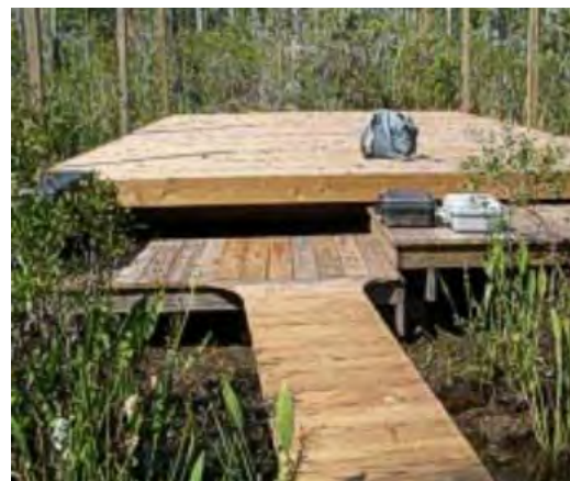
Flat docks with no roof or wall structure. Source: Seaside Water Trail Camping Platform Feasibility .
