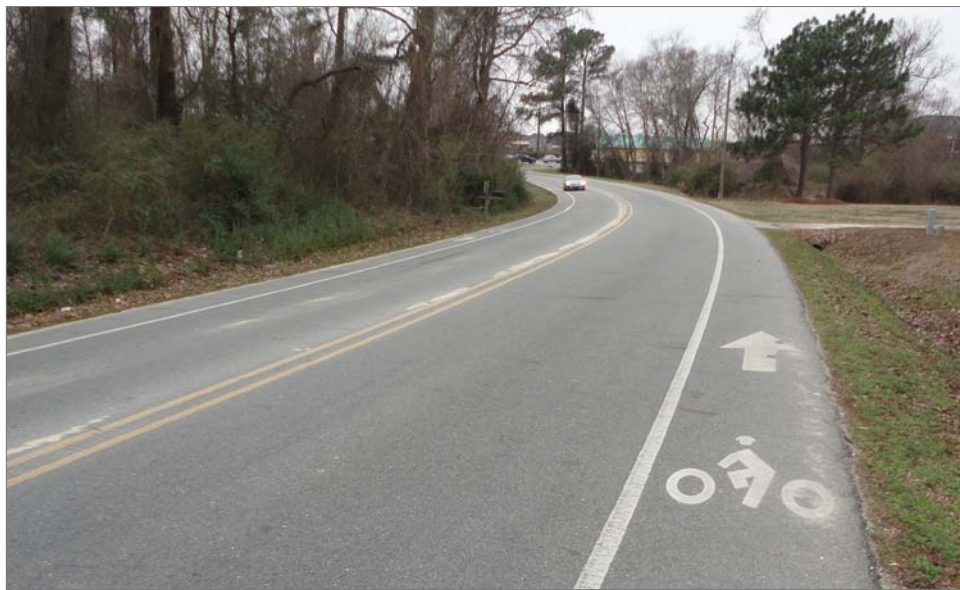
Bike lane on Harding Drive in Goldsboro. See Appendix A, page A-30 for bike lane design guidelines.
