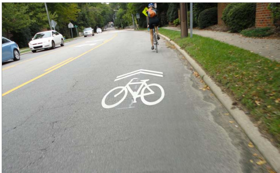
Sharrows in Raleigh, NC. See Appendix A, page A-26 for sharrows design guidelines.
