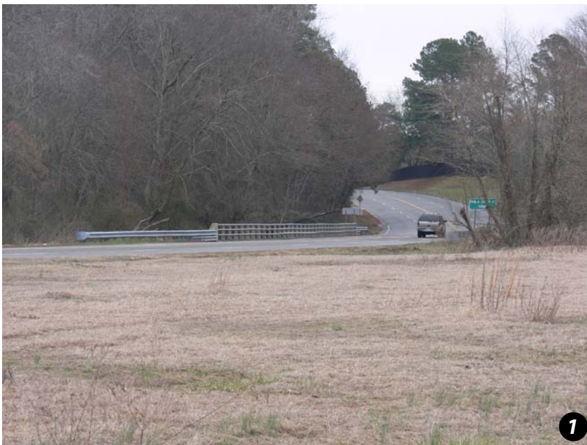
The City-owned parcel on south side of Elm is an ideal location for the trailhead. The HAWK signal would be located near this location across Elm Street.
