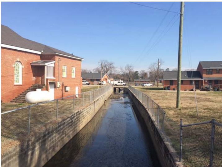
Portion of the “Ditch” with concrete channel through a public housing area at Elm Street.
