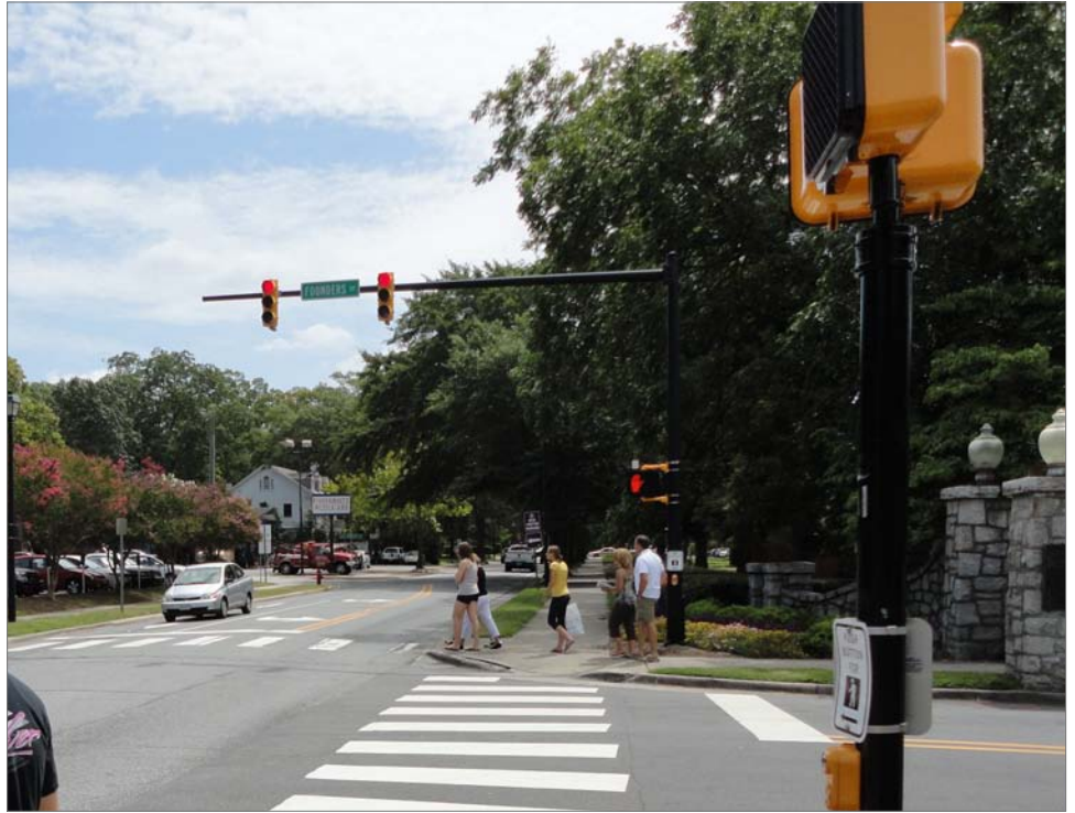
Countdown signals (and marked crosswalk) in Greenville, NC
